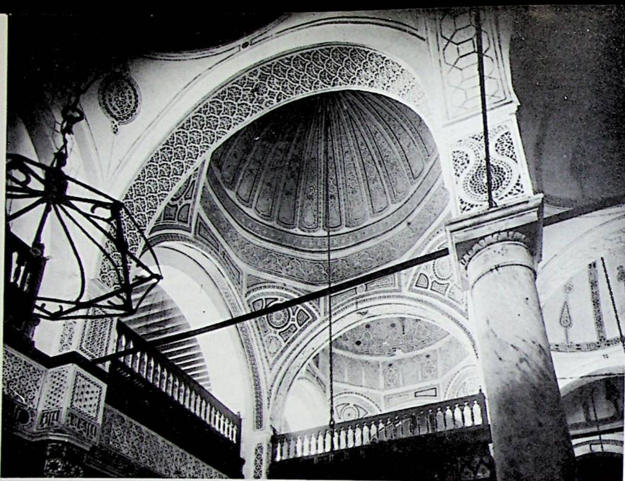
Plaster work on the ceiling of Ahmed Pasha Mosque in Tripoli.
